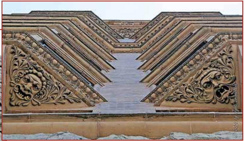
Figure 2 – Views of projecting bays on Chicago skyscraper buildings in response to the Chicago Building Codes of 1905.
