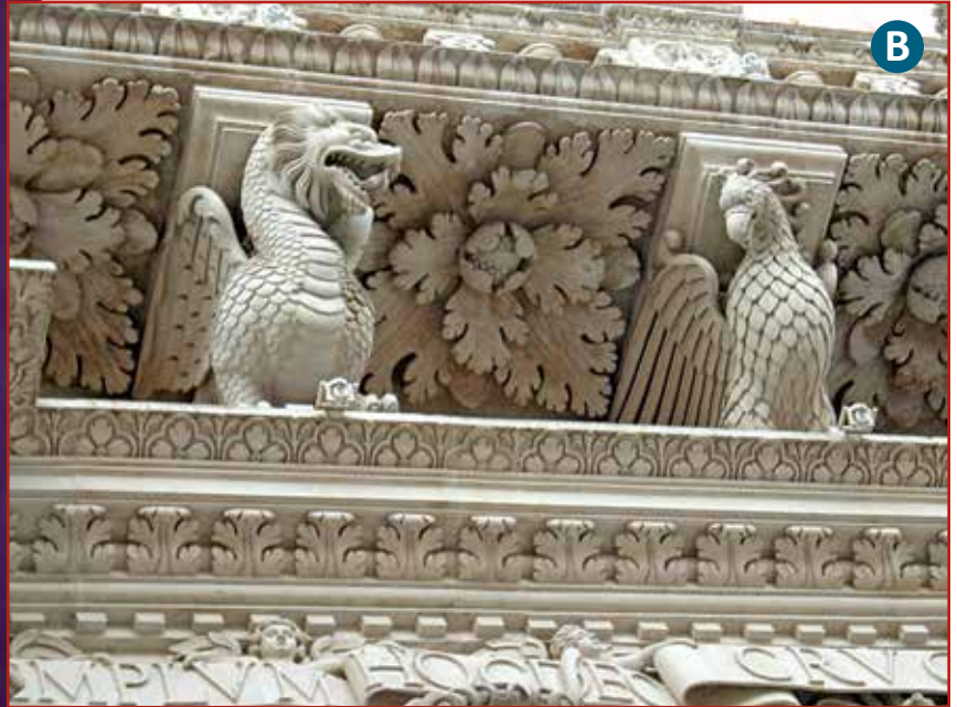
Figure 7 – Figure 7A shows a photo-elastic model for a flying buttress structure indicating the load demands. 15 Figure 7B shows a simpler example of integral ornamentation in structure with the use of figural elements to act as brackets supporting the balcony above.
