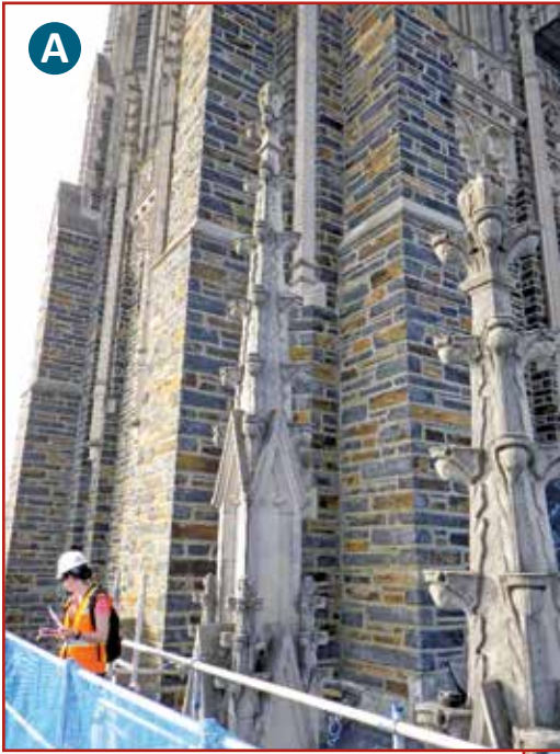
Figure 11 – Large stone finials used at the terminus of the wall and towers to limit water infiltration at the roof and wall interface were utilized as designed ornaments at collegiate buildings.
