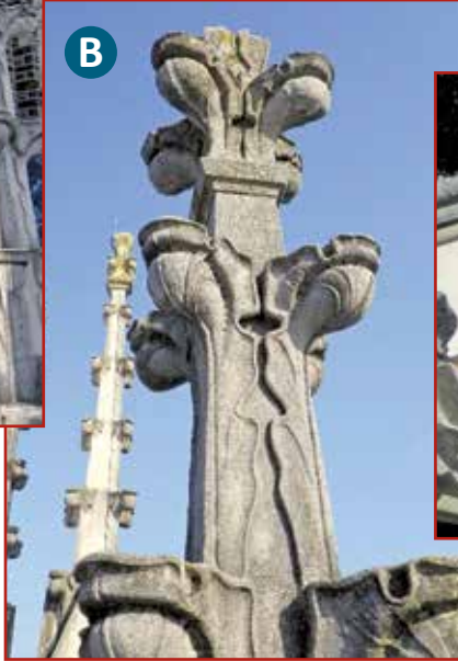
Figure 11 – Large stone finials used at the terminus of the wall and towers to limit water infiltration at the roof and wall interface were utilized as designed ornaments at collegiate buildings.
