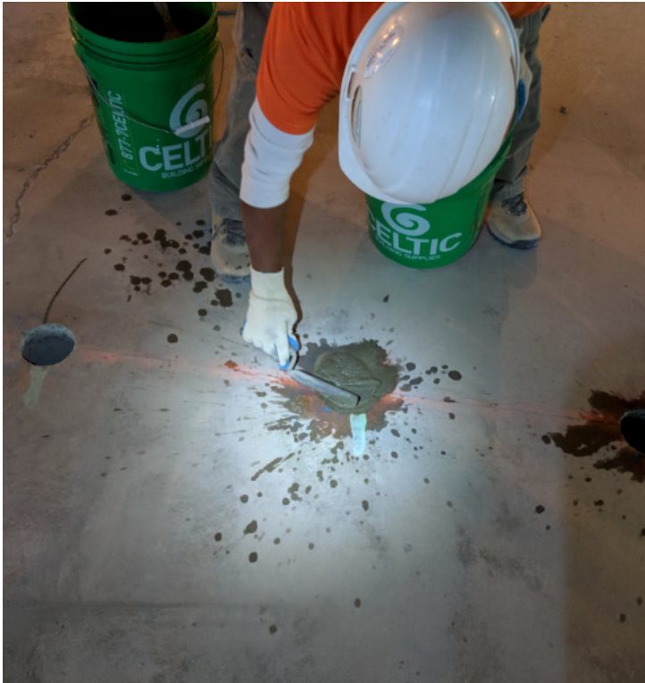
Figure 7. Non-shrink grout placement in core holes.
