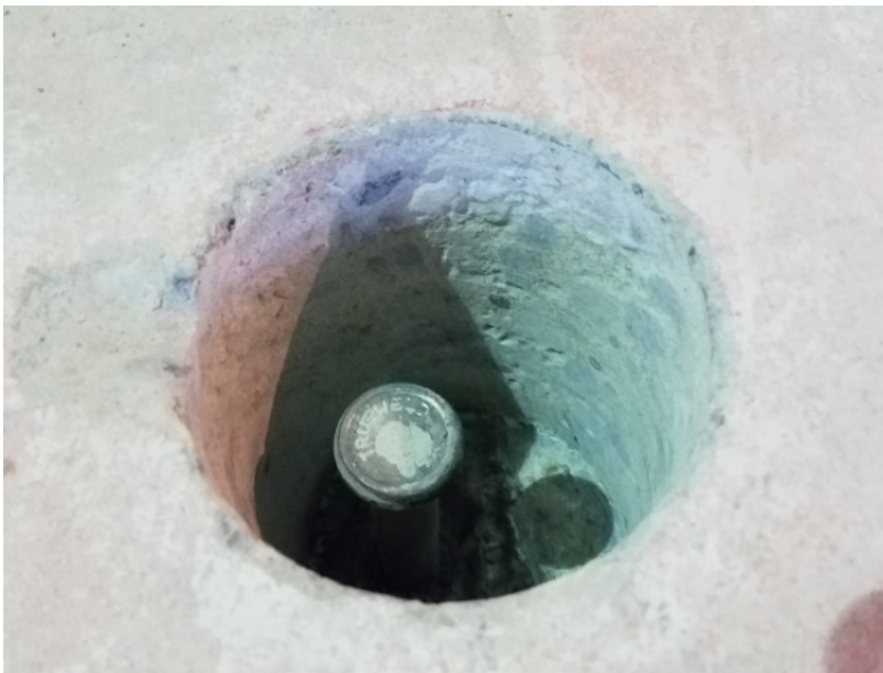
Figure 6. Headed shear connector welded to top flange of existing steel beam.
