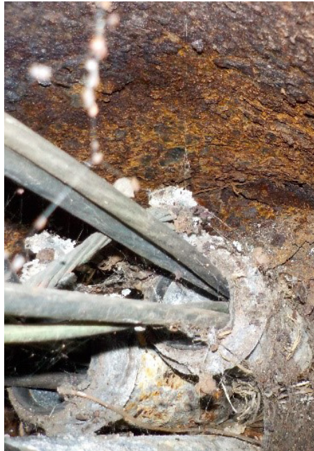
Figure 13. Interior view of subject pole.
