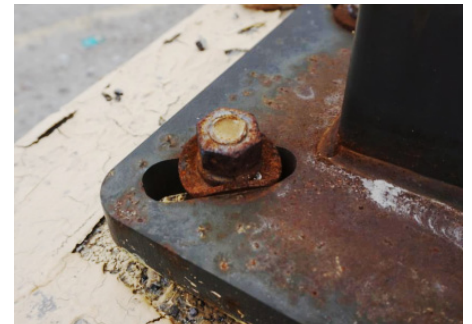
Figure 8. Deformed washer.
