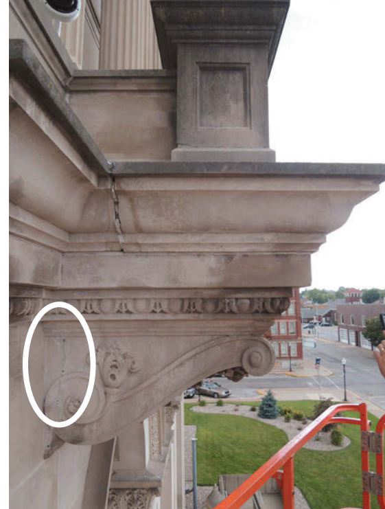
Figure 2. Epoxy repair at cracked cantilevered corbel.
