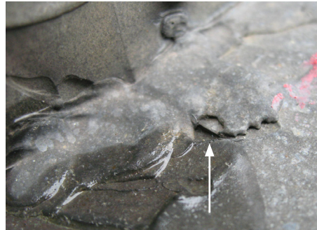
Although the holiday in this lapped, riveted, and soldered seam is only about 1/16" wide, it offers a direct path for significant water entry, especially if the gutter outlet tube should clog and a head of water form.
