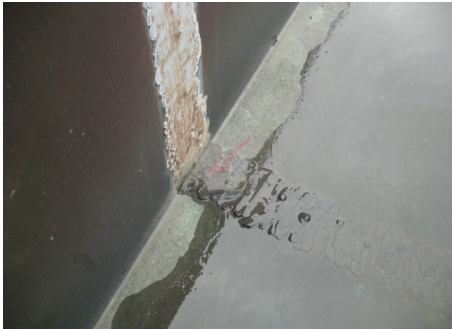
Although the holiday in this lapped, riveted, and soldered seam is only about 1/16" wide, it offers a direct path for significant water entry, especially if the gutter outlet tube should clog and a head of water form.
