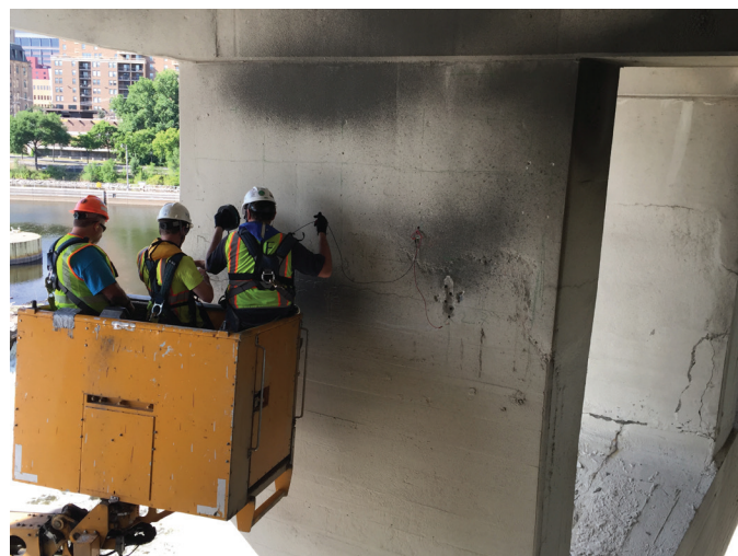
Fig. 2: Engineers utilizing three under-bridge inspection units for close-up bridge inspection and sounding during the Phase 1 bridge inspection (photograph by WJE).
