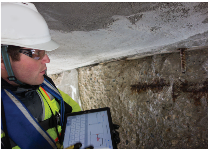
Fig. 3: Bridge inspector recording notes utilizing proprietary iOS-based tablet inspection software (photograph by WJE)
