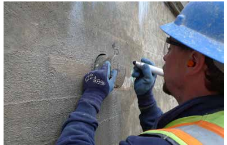
Figure 2: Concrete core sampling for corrosion testing
