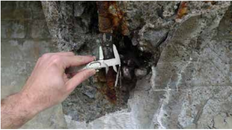
Figure 1: Deformed square cross-section reinforcing bar
