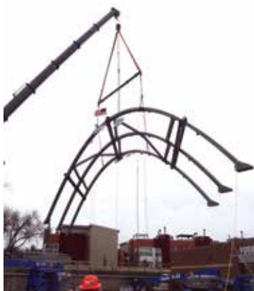
Figure 4. Lifting the arch assembly.
