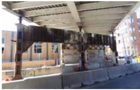
Figure 2. The elevated bridge structure.
