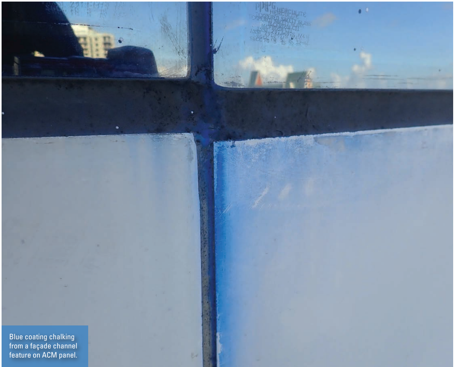
Sealant failure and blue coating chalking at a façade channel feature.
